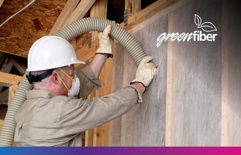
Dry Dense-Packing Wall and Floor Assemblies
