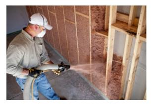
Only Greenfiber FRM Insulation may be used as a fireblocking material in the the SANCTUARY Two-Hour Firewall, UL-U370 assembly. This product can be identified by it's proprietary a terracotta color.
