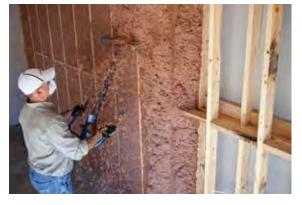
Only Greenfiber FRM may be used as a fireblocking material in the UL370 assembly. This product can be identified by it's proprietary a terracotta color.
