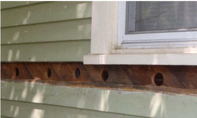
2. Using a hose clamp, attach the 1 to 1 ½ - inch reducer nozzle to the insulation blowing machine hose.
