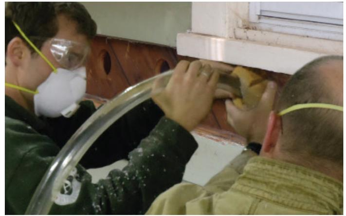
6. Insert cut end of the tube through the filter into the 2 ½-inch drilled hole and feed to within 6-inches of the top of the stud cavity. Note any fire stops or other obstructions. Drill additional holes as needed if obstructions are present.
