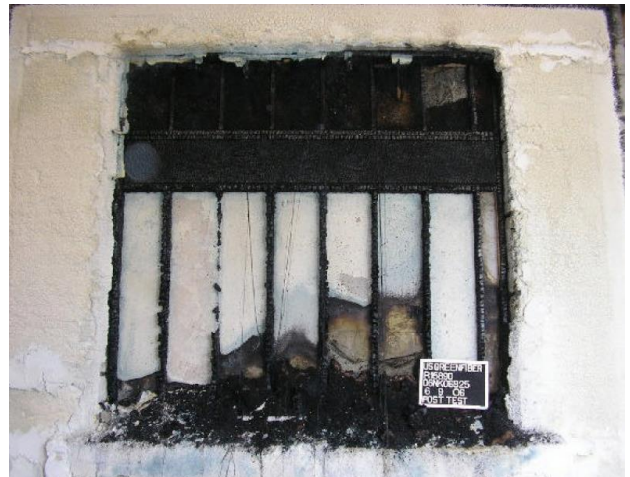
Exposed Surface – Post-Test Photo
